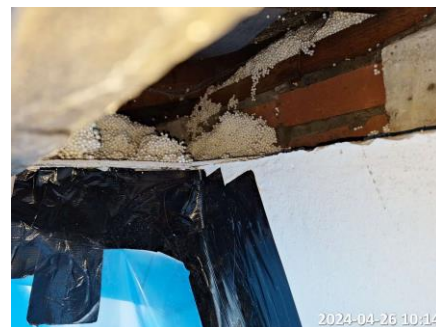
2/3. AIB soffits over neighbours property left in place
