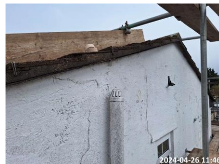
4/3. Undercloaking left in place
